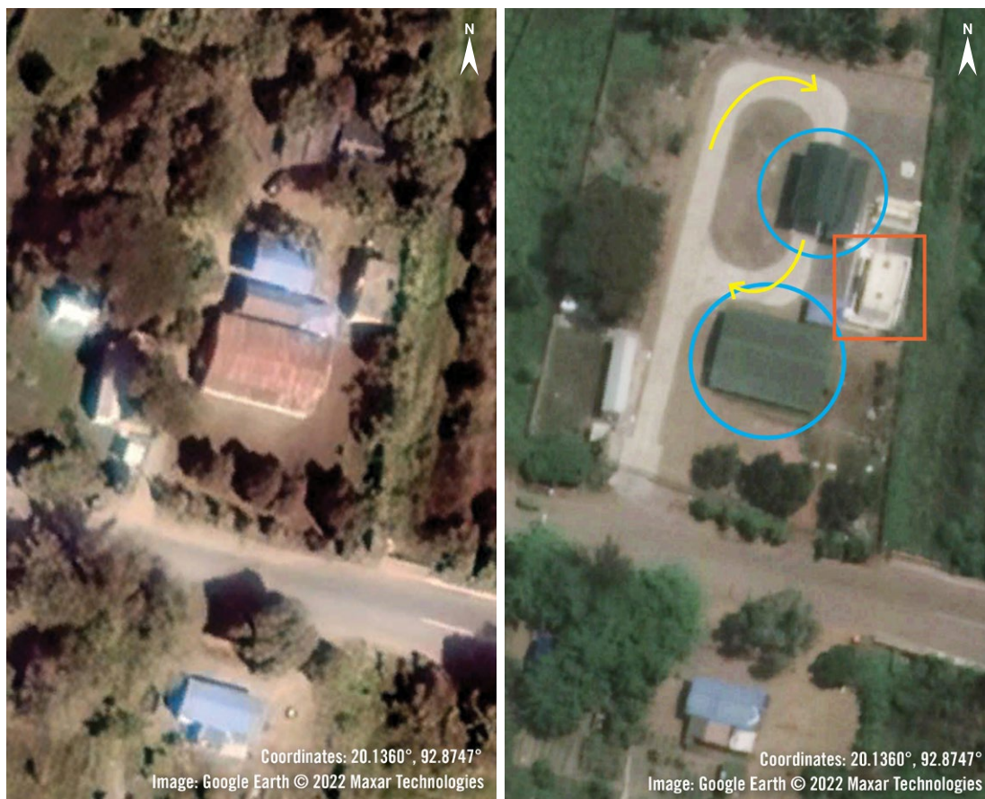
Sittwe, Myanmar: Satellite imagery shown above is an example of the changes to fuel storage facilities at airports where NEPAS began delivering fuel. In 2016 (left image), imagery shows the old fuel storage area at Sittwe airport. In 2018 (right image), the road through the facility appears expanded, paved and redesigned in a circular pattern, allowing trucks to move through easily. A new building was constructed, and another building appears to have an updated green roof – both highlighted with blue circles. A fuel storage tank – highlighted in orange – appears updated with new pipes.
