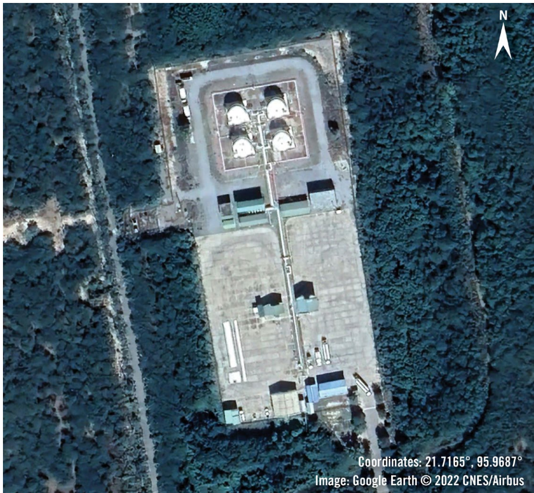
NEPAS storage facility at Mandalay airport.
