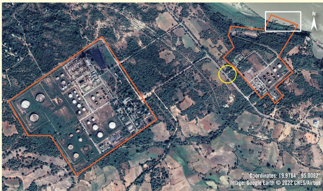
Mann Thanbayakan Petrochemical Complex, Myanmar: Satellite imagery shows the Mann Thanbayakan Petrochemical Complex, located approximately 20 kilometres south of Magway, Myanmar. The refinery has a complex area inland and one along the shore – highlighted in orange. At the shore of the river, barges are often seen in satellite imagery in the area highlighted with a white box. Many fuel trucks have also been seen over time at the entrance to the complex along the shore – highlighted with a yellow circle.
